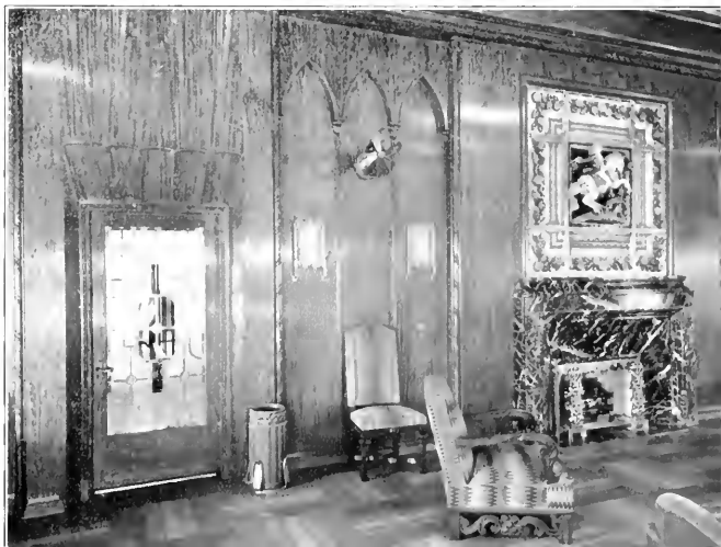
Detail of Bulkhead, Fireplace, and Door in Smoking Room
